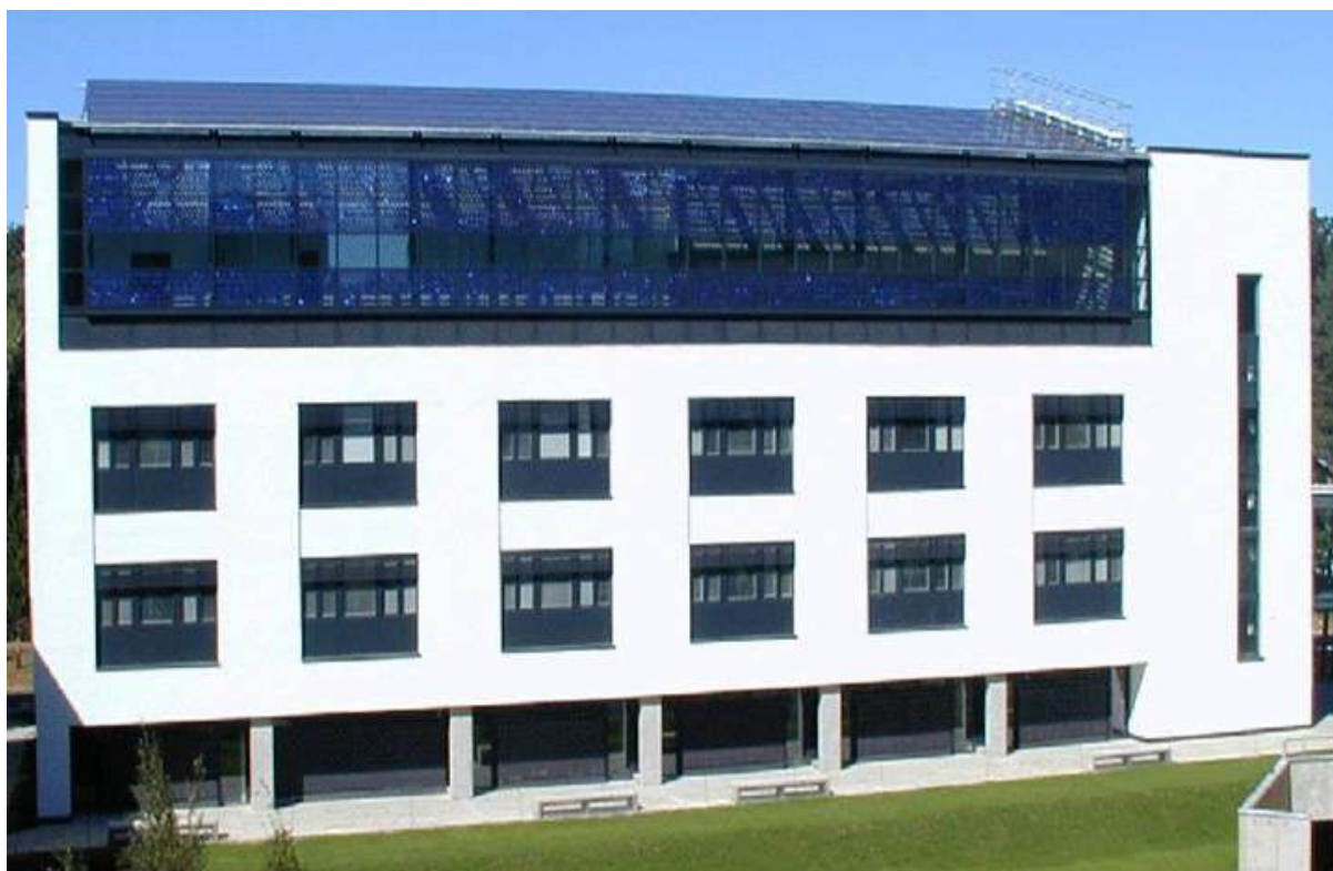
Figure 1 Solar panels installed at the Zuckerman Institute for Connective Environmental Research (ZICER) Building
